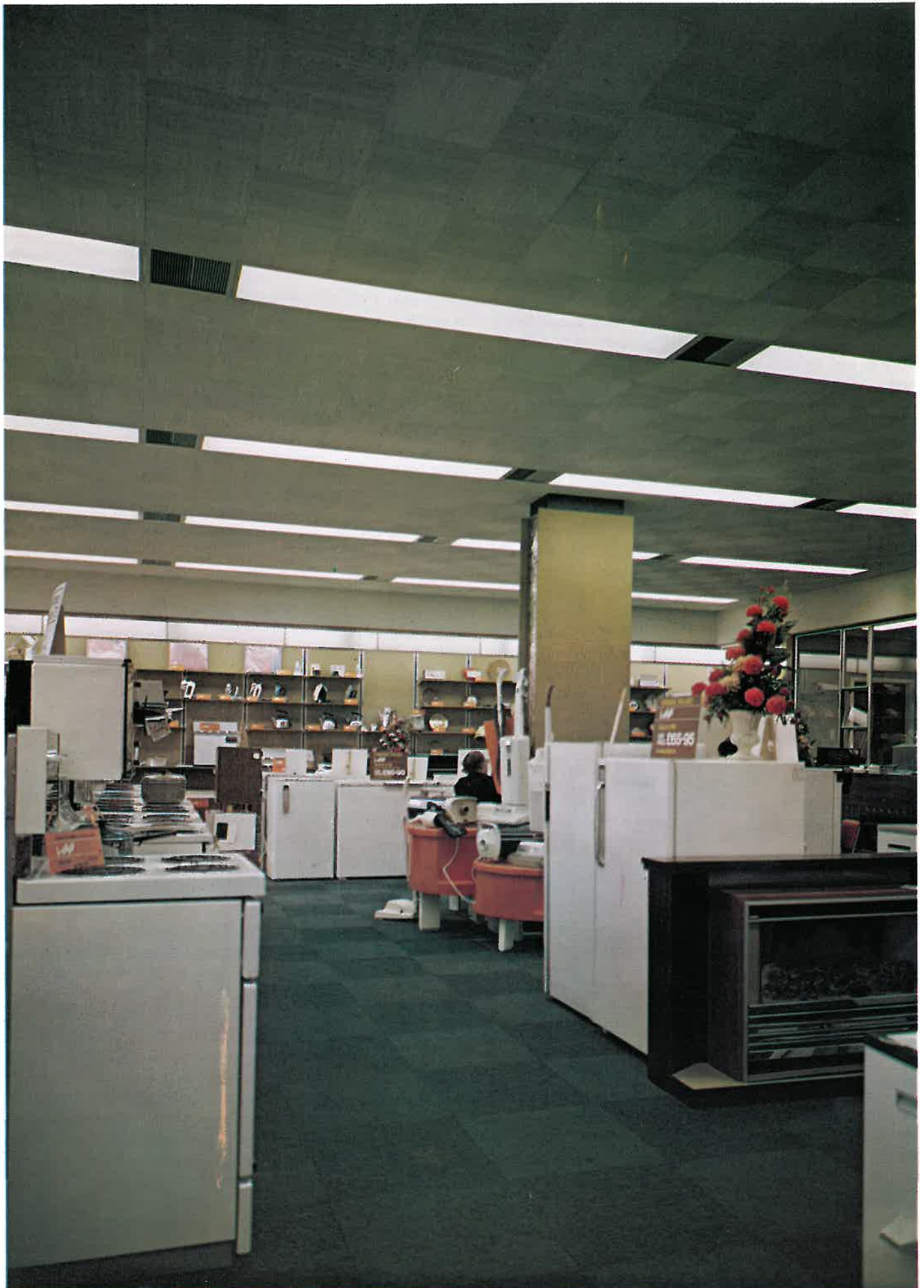
First installation of the Arena system is in the London Electricity Board's new showroom at Poplar, London. Since they are used for air input only, the grilles are mounted with their blades running across the lines of lighting units.
